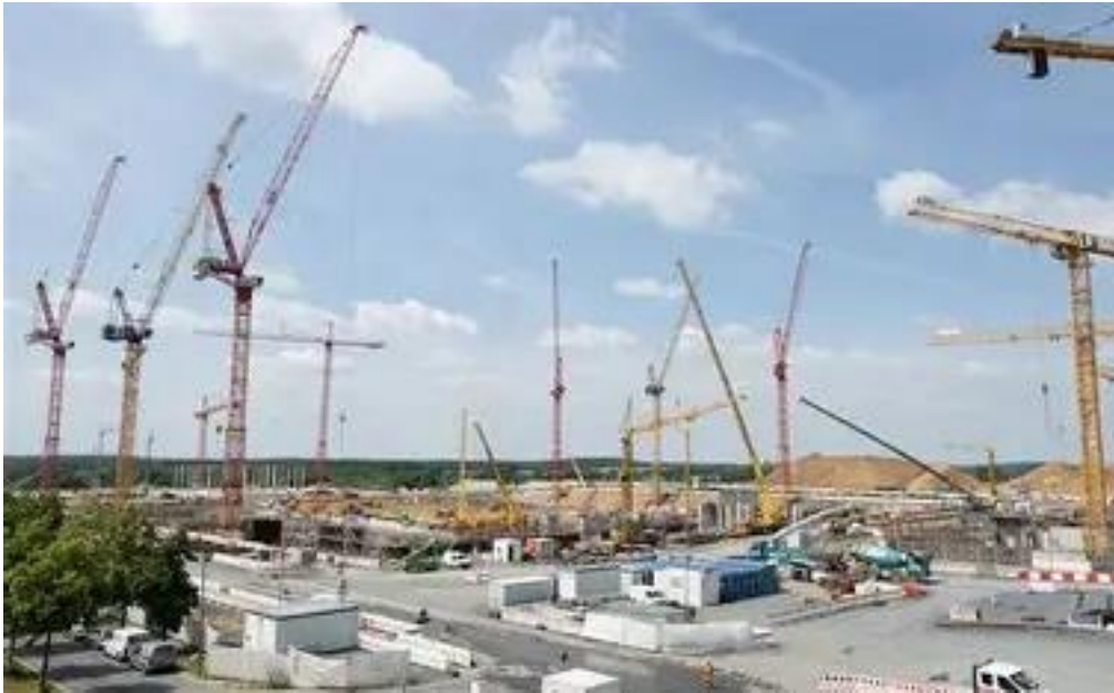
ESMC Drezno-Silicon Saxony, plac budowy
